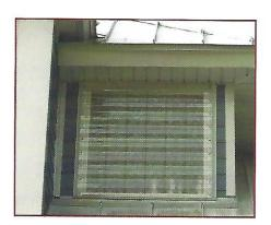
by GE. Easy accessibility to windows and doors is needed when using storm panels, they don't install easily from a ladder. Storm panels work fine for protection
